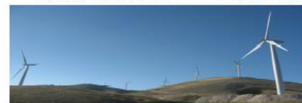
San Gregorio Magno wind farm
